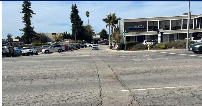
Old Utility Trench Repairs and Faded Striping
