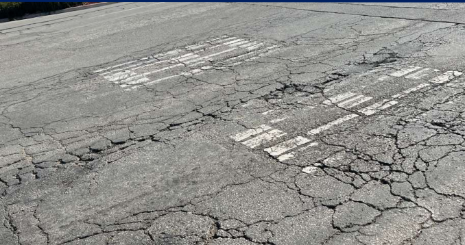
Depressions and Uneven Pavement
