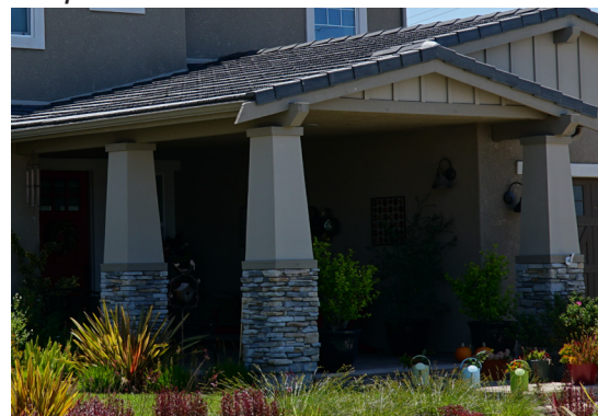
Example of Columns
