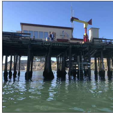
PHOTO 3 WHARF BELOW CRANE
