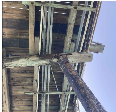
PHOTO 7 UTILITIES BELOW DECK
