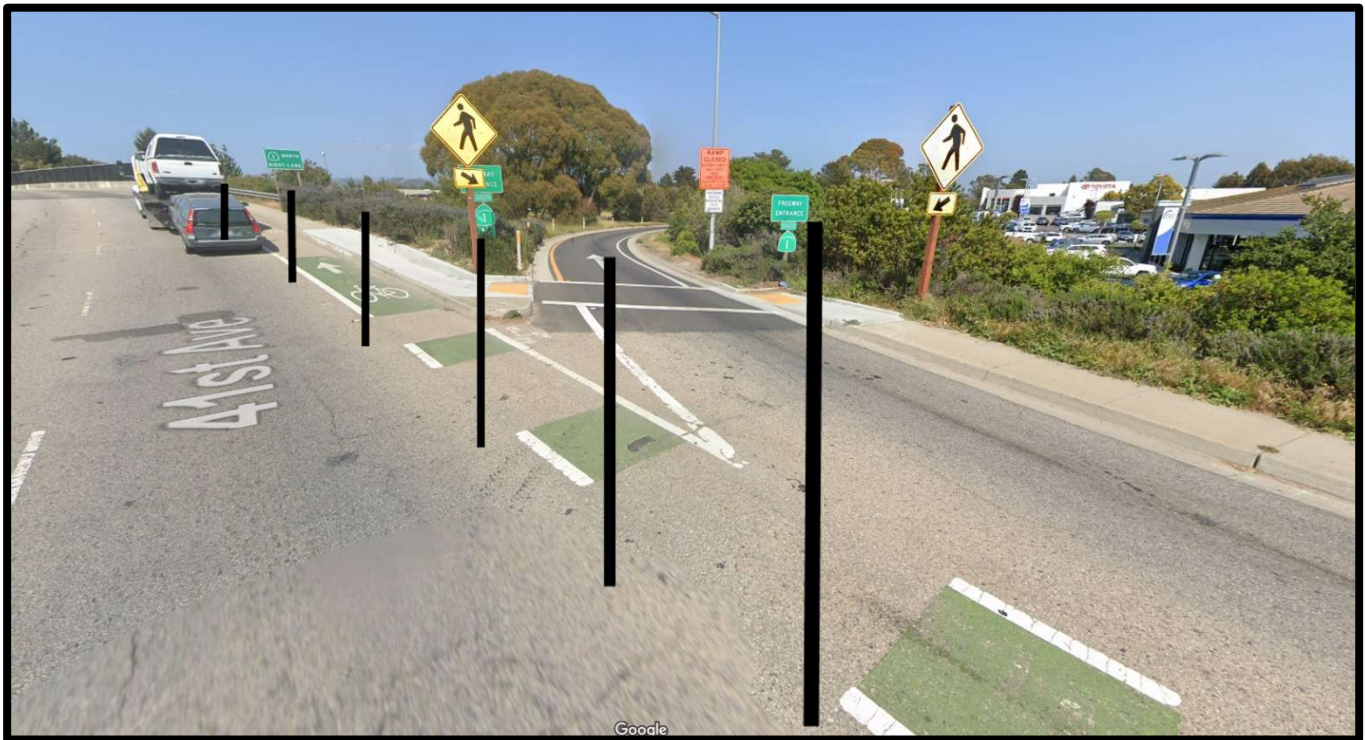
Proposed location of physical barrier on 41 st Avenue at Highway 1 southbound on-ramp
