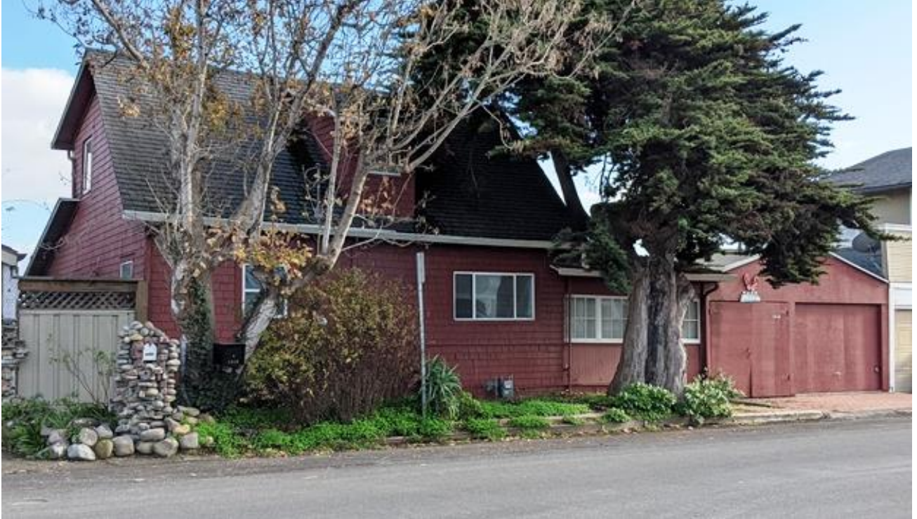
Front (Prospect Avenue) Façade. Viewed facing southeast. January 2020. (Photo by Leslie Dill)
