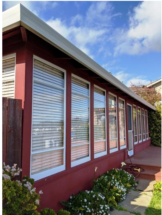
East Façade of Wrap-around Wing. Viewed facing northwest. January 2020. (Photo by Leslie Dill)
