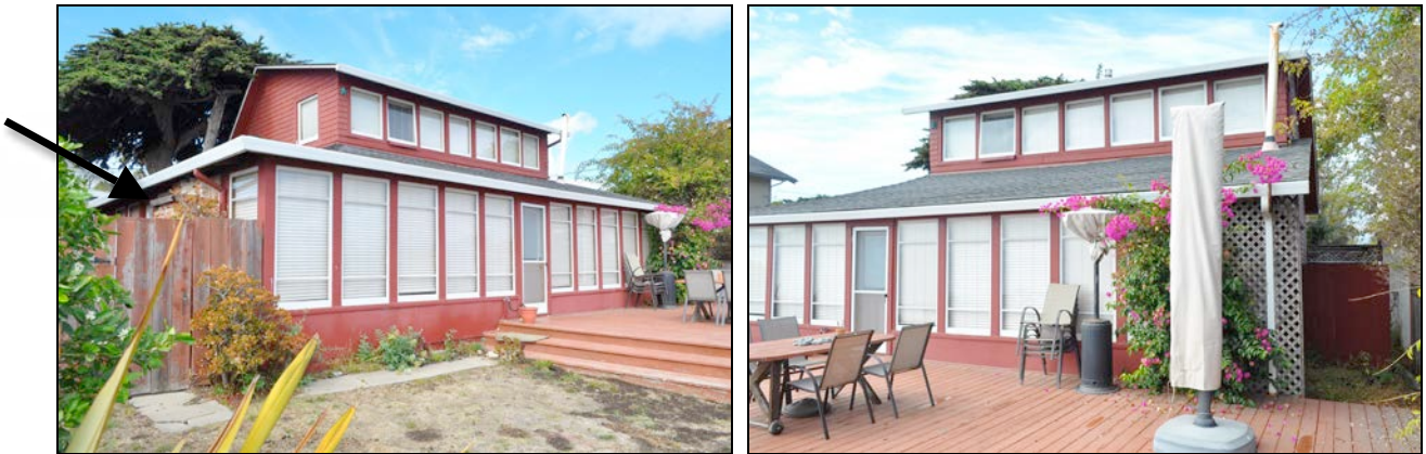
Figures 3 and 4. Left image shows the asymmetrical roofline of the Monterey Bay (east) elevation. The clipped brick chimney is on the south elevation (arrow). Right image details the banked windows of the east elevation.
