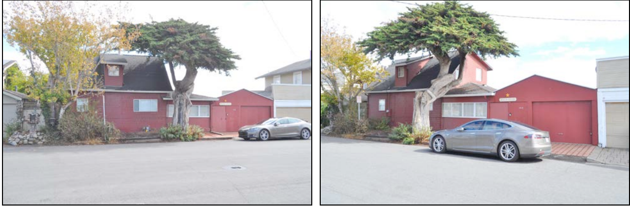
Figures 1 and 2. Left image shows the Prospect Avenue (west) elevation, as viewed from the street. Right image details the west elevation, showing the false-front, gable-roofed garage.
