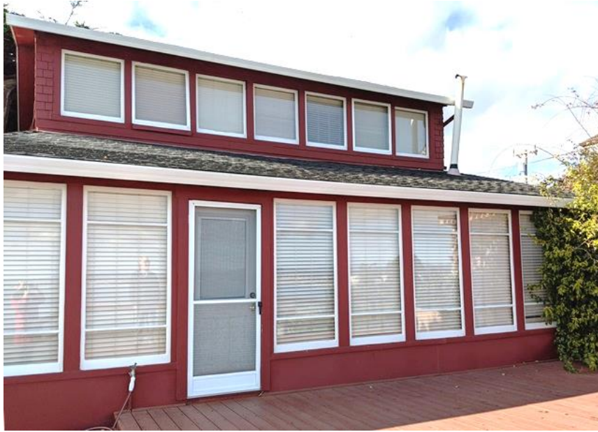
Ocean-facing Façade. Viewed facing northwest. January 2020. (Photo by Leslie Dill)
