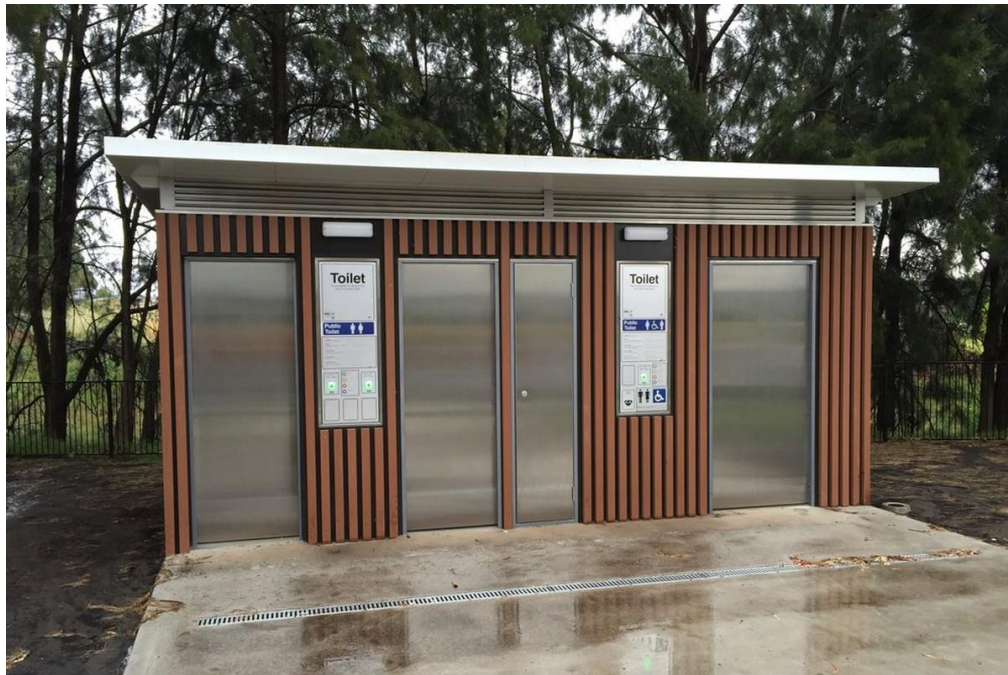
Figure 3. Exeloo triple cubicle restroom exterior
