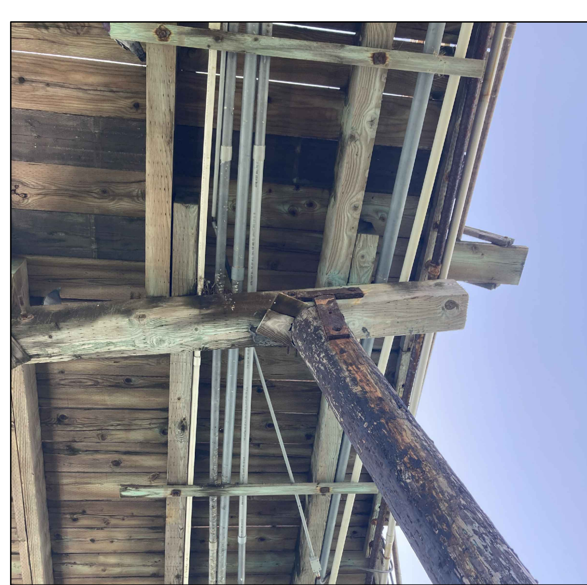
PHOTO 7 UTILITIES BELOW DECK
