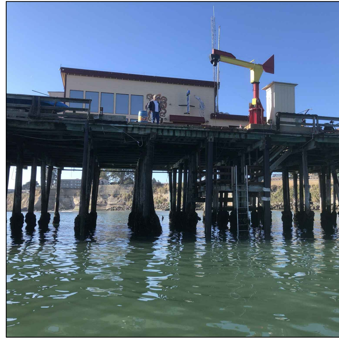
PHOTO 3 WHARF BELOW CRANE
