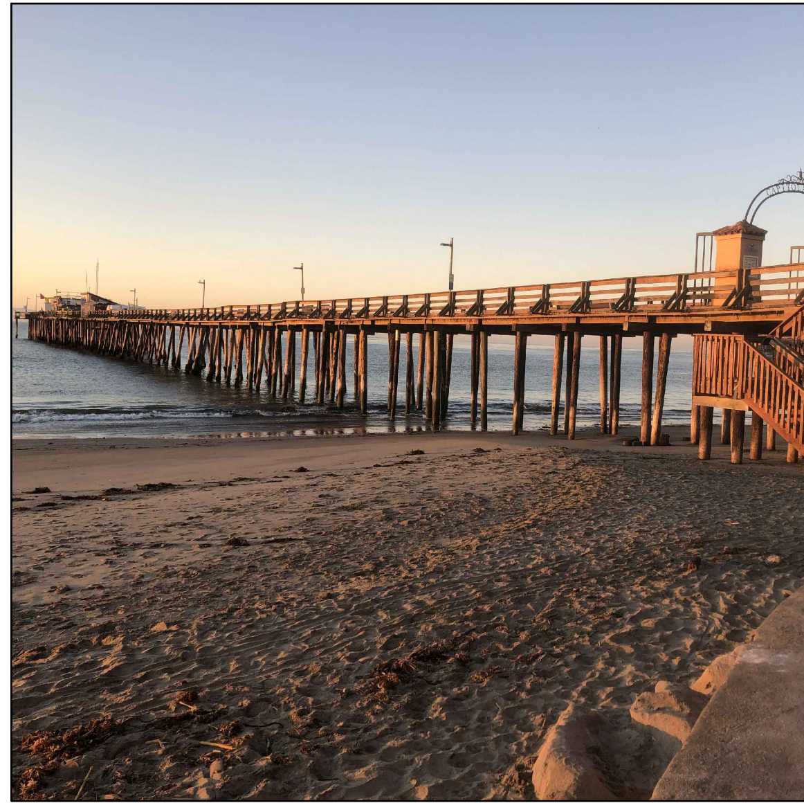
PHOTO 1 OVERALL VIEW OF WHARF
