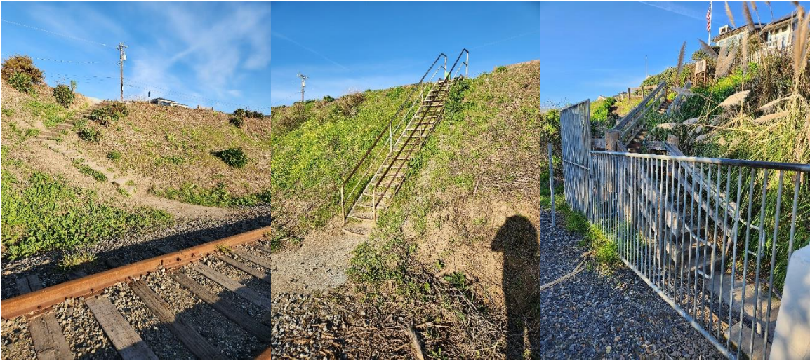
Figure 2. Stairways Maintained by the City
