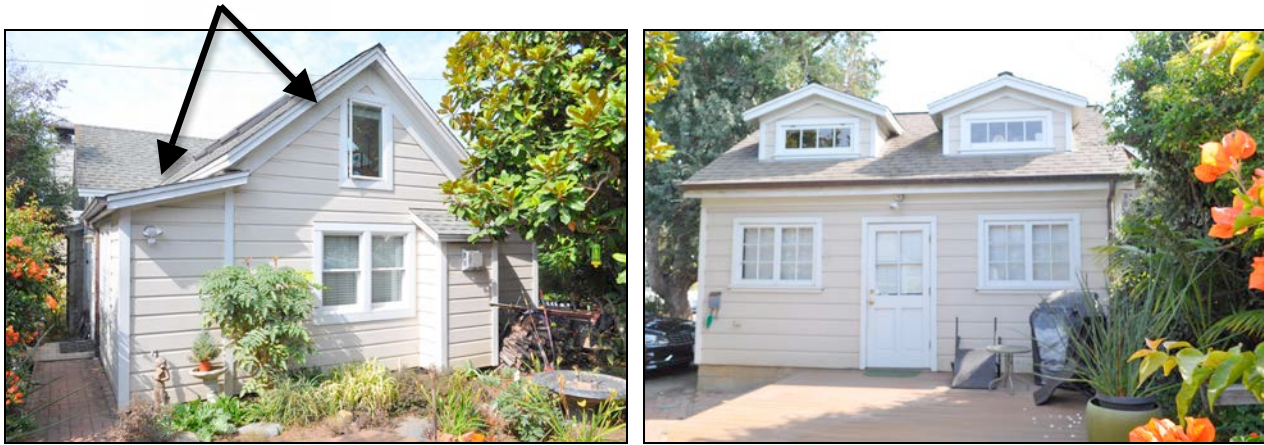
Figures 3 and 4. Left image shows the rear (east) elevation, with arrows indicating the large, circa-2000 addition installed behind the side gable roof. Right image shows the relocated garage.
