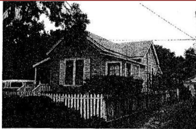
112 Central Avenue Vernacular Cottage c. 1900
