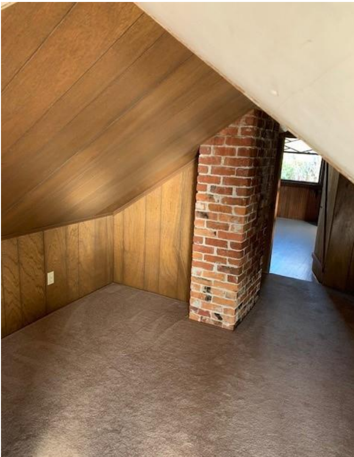
Central attic third-story space.
