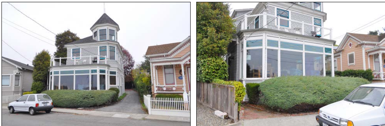
Figures 1 and 2. Left image shows the front (west) elevation, as viewed from the street. Right image details the front porch enclosure on the west elevation.
