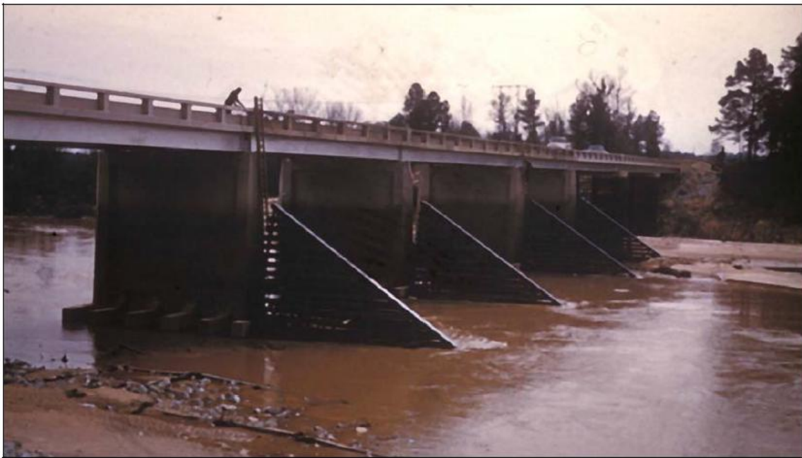
Figure 9. Photo of timber debris fins with sloping leading edge.
