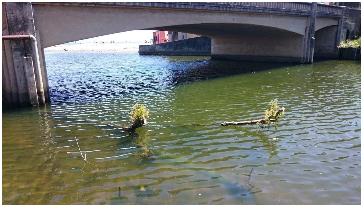
Figure 6. Photo, Looking Downstream, Stockton Avenue Bridge
