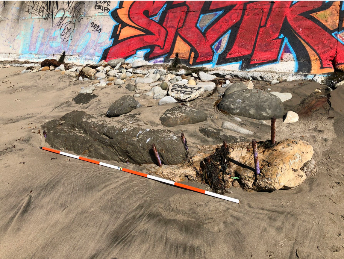
Photo 2: Close up of shotcrete, bedrock, rebar debris to be removed - 26 May 2020
