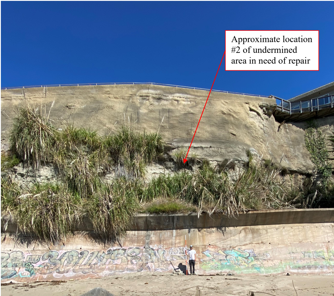
Photo 4: 4800/4820 Opal Cliff Drive Property Line View - 26 May 2020
