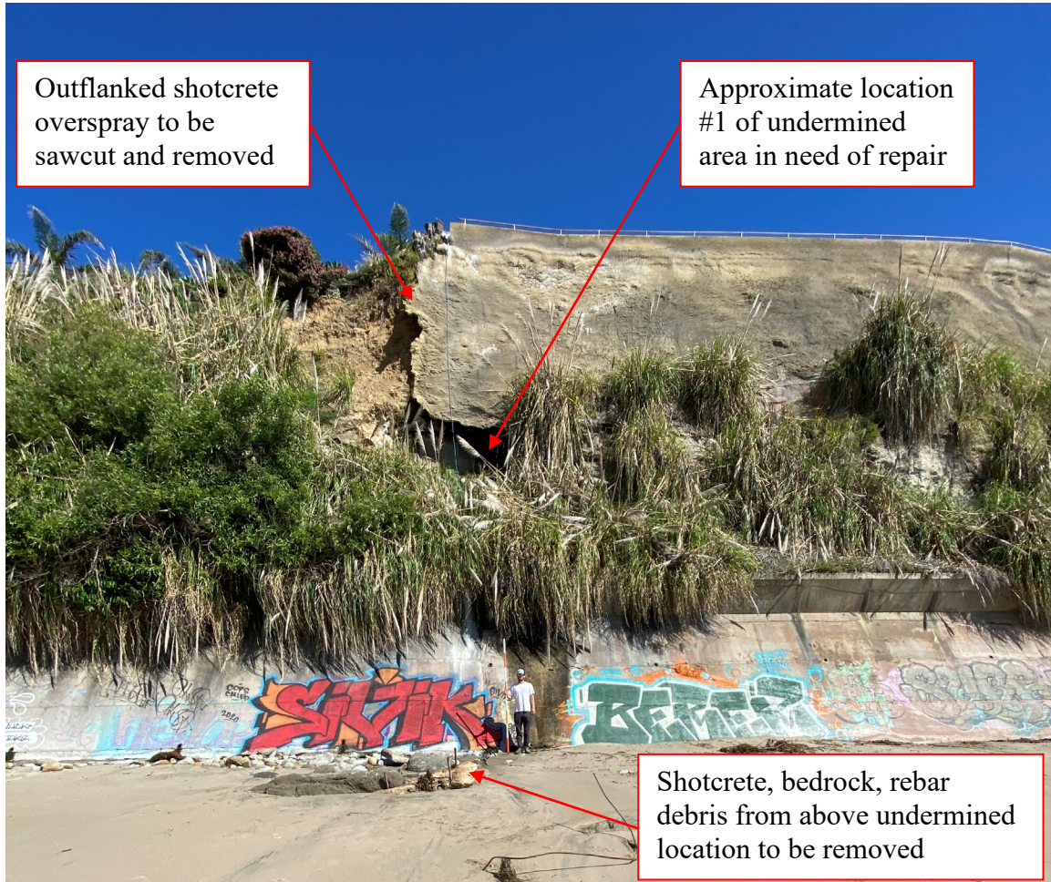
Photo 1: 4800/4790 Opal Cliff Drive Property Line View - 26 May 2020
