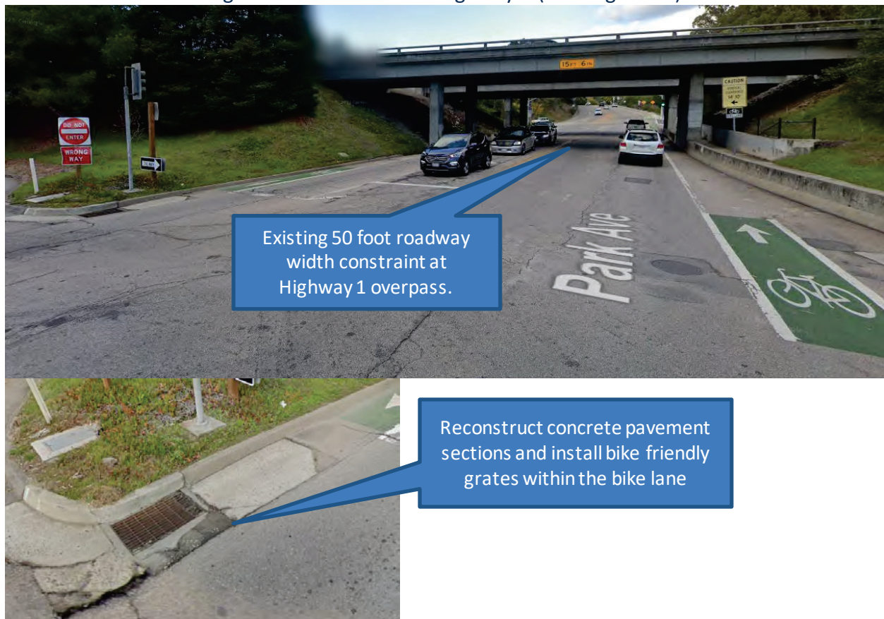
Figure 2: Park Avenue at Highway 1 (Looking North)
