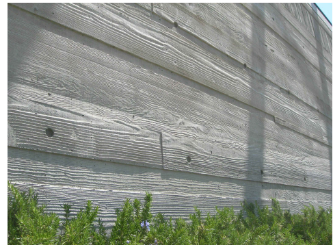
BOARD FORM FINISH CONCRETE SEAT WALL
