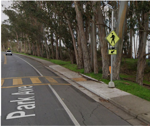
Flashing beacon pedestrian crosswalk at Cabrillo
