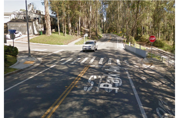
All way stop control and crosswalk at Coronado
