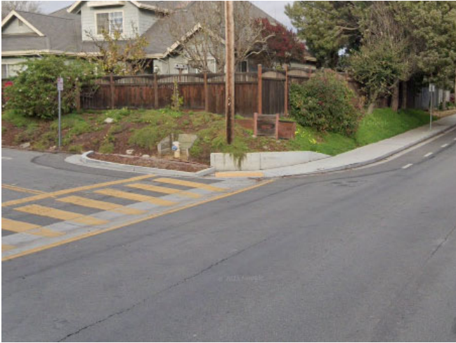
Sidewalk and striped crosswalks on north side
