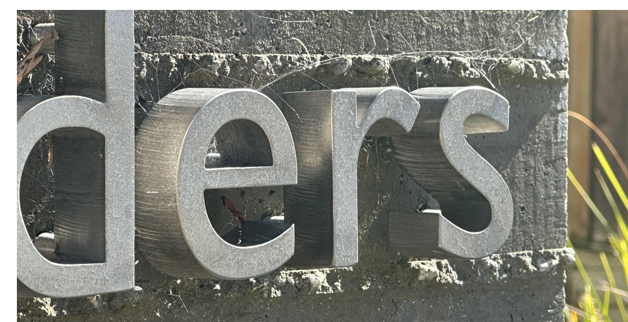
STAINLESS STEEL LETTER ON STANDOFFS OR CAN BE INTERNALLY ILLUMINATED
