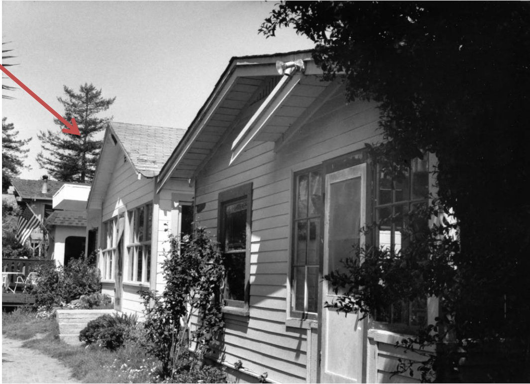
Figure 5. View looking north along the residences' west-facing elevations. An arrow indicates the subject property. Note that the rear entrance utilized a series of concrete stairs and no porch rail ( Courtesy: Charles Rowe, Old Riverview Historic District, National Register of Historic Places Registration Form (listed, 1988)).
