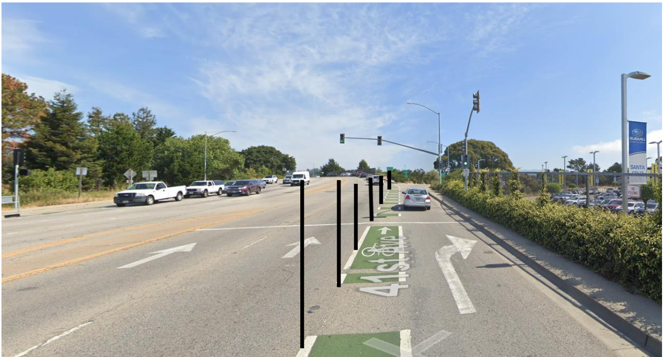
Figure 1. Location of physical barrier on 41 st Avenue approaching Highway 1 southbound on-ramp
