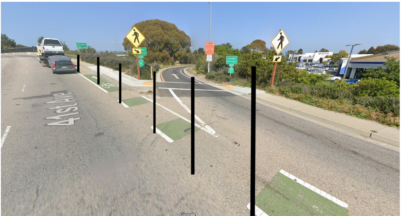
Figure 2. Location of physical barrier on 41 st Avenue at Highway 1 southbound on-ramp
