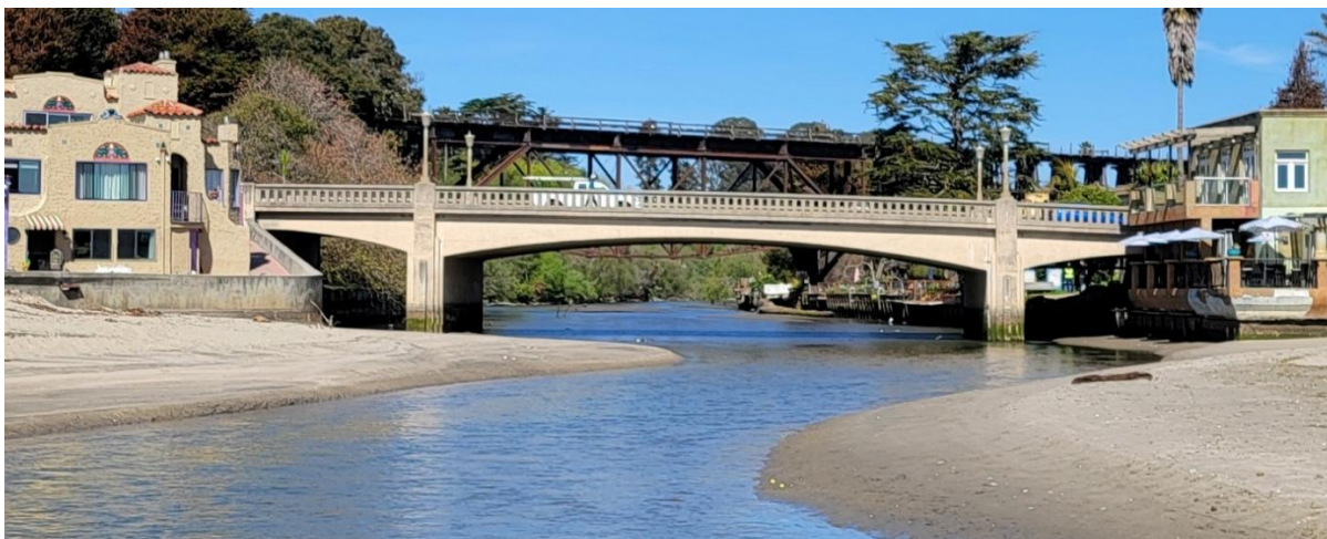
Figure 1: Stockton Avenue Bridge Looking Upstream
