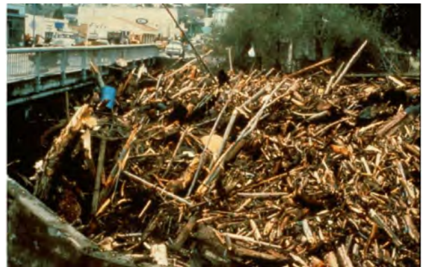
Figure 8 Logjam Upstream of Soquel Drive Bridge after January 1982 Storm
