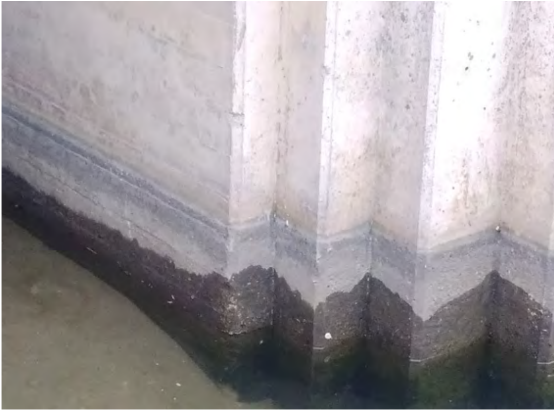
Photo 1. Close Up Photo of OWHM on the south pier of Stockton Bridge (5/14/2024).
