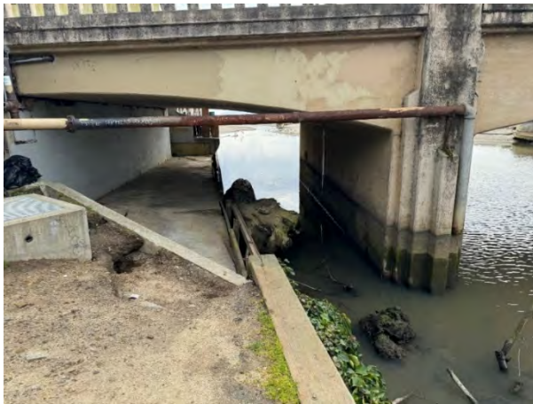
Figure 7 Collapsed Sidewalks
