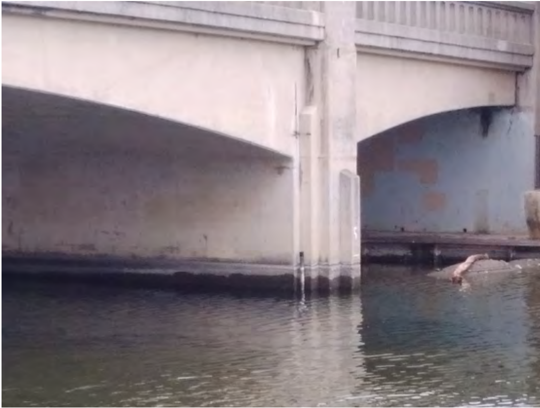
Photo 3. OHWM on the north pier of Stockton Bridge (5/14/2024).
