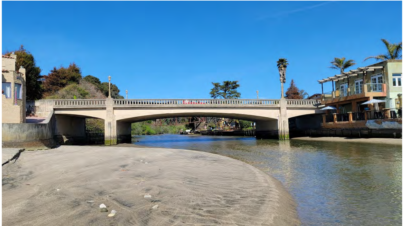
Figure 2 Western View of Stockton Avenue Bridge
