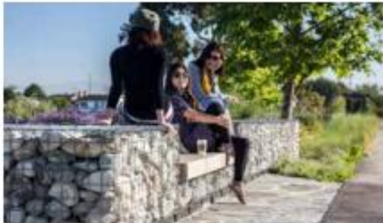
Gabion retaining and seat wall with integrated bench. (Photo by: SWA)
