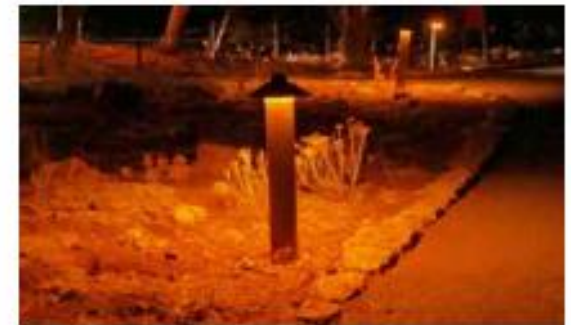
Bollard lighting options are appropriate along trails. (Photo by: Michael Quinn)
