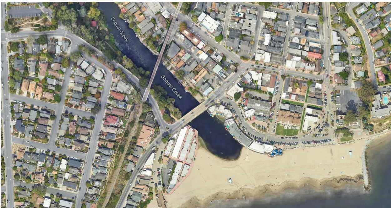
Aerial photograph of Soquel Creek and Stockton Avenue Bridge
