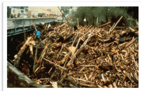
Figure: 1982 Debris Accumulation upstream of Soquel Drive Bridge.
