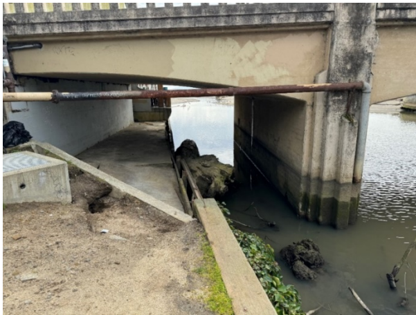
Figure 7 Collapsed Sidewalks
