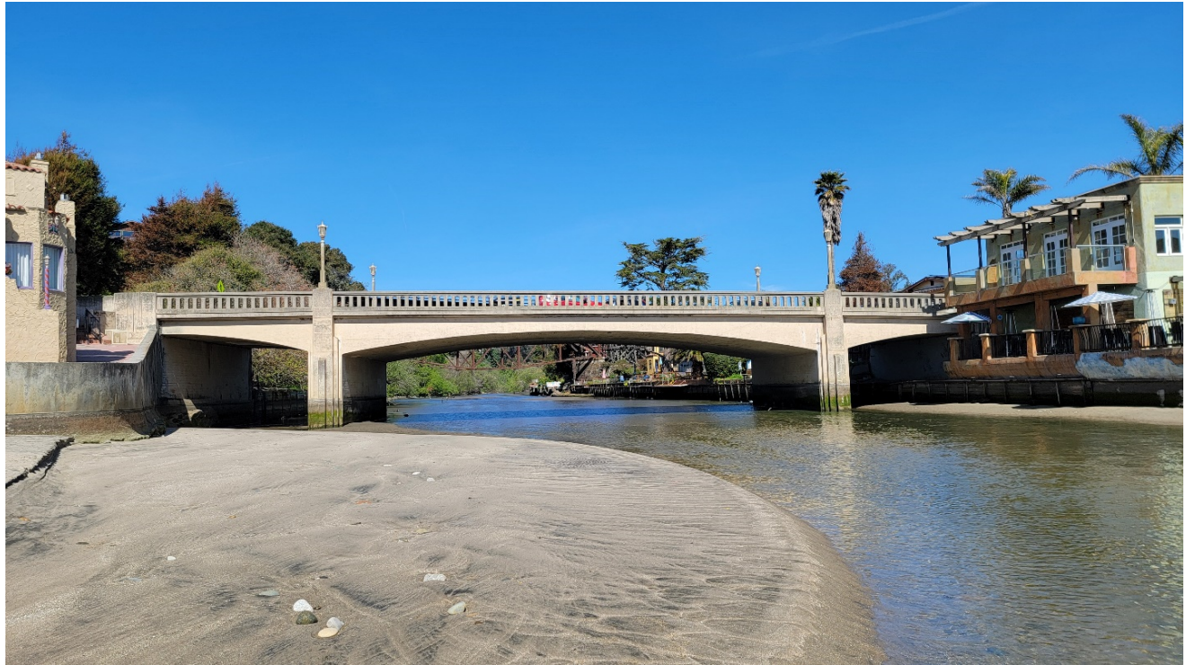
Figure 2 Western View of Stockton Avenue Bridge
