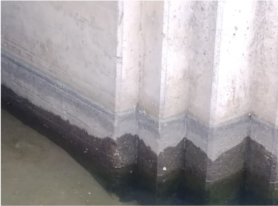
Photo 1. Close Up Photo of OWHM on the south pier of Stockton Bridge (5/14/2024).
