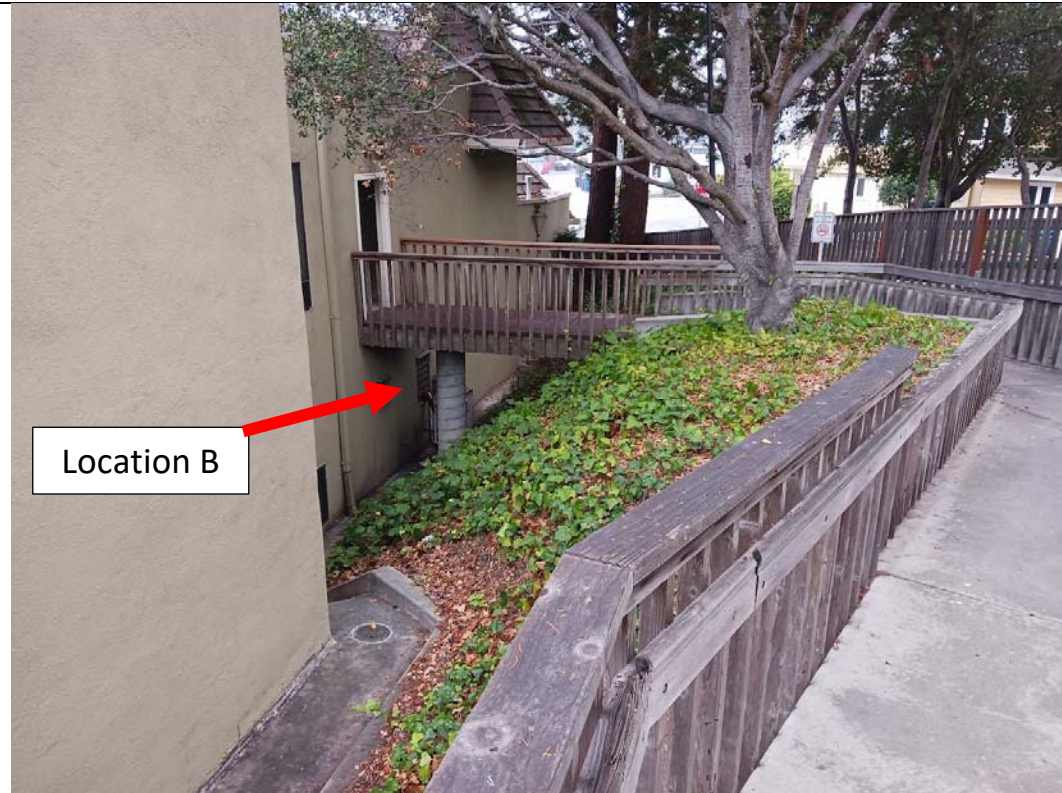
Location B – Electrical Room
