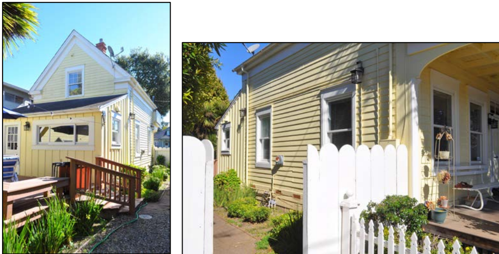
Figures 3 and 4. Left image shows the rear (west) elevation, with shed roofed rear addition. Windows in the rear addition have been replaced in original and new openings. Right image details the south elevation. Original wood sash windows have been replaced.
