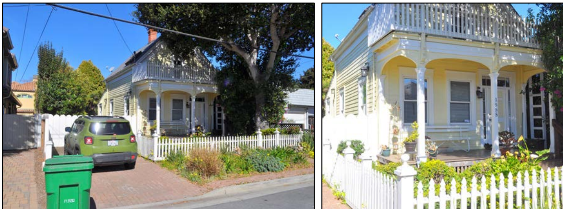
Figures 1 and 2. Left image shows the front (east) elevation, as viewed from the street. Right image details the front porch, which was replaced in the 1970s and the porch roof converted to a deck.
