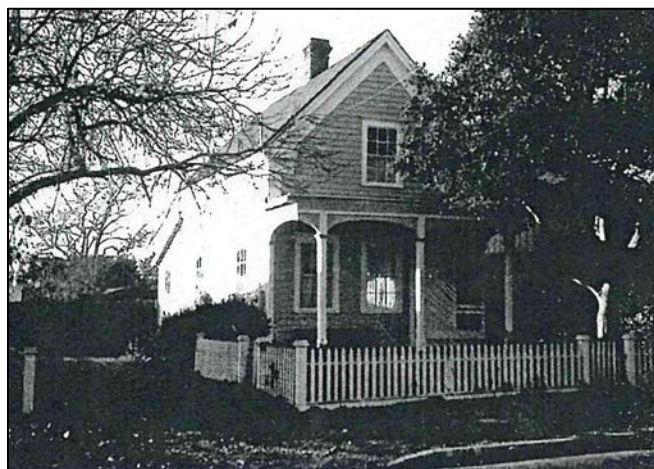
Figure 7. 1975 Assessor's photograph showing the second-story, gable-end window and the replaced front porch.
