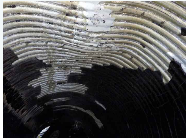
Photo 18. Station 3+54; signs of minor corrosion on deformed bulge.
