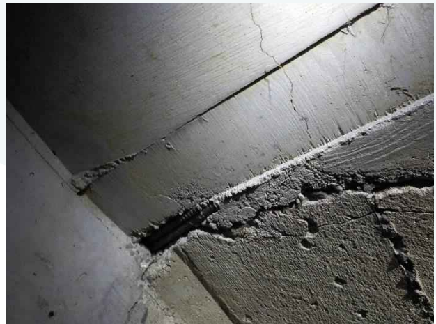
Photo 8. Station 0+54; exposed reinforcement on ceiling at concrete joint.
