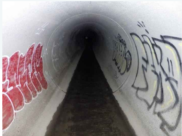
Photo 35. Station 1+25; RCP section of segment was in good condition.
