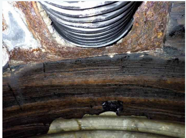
Photo 28. Station 3+84; minor corrosion of metal at lateral break in site.
