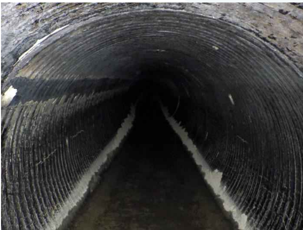
Photo 21. Station 0+00; signs of coal tar deterioration along pipe.
