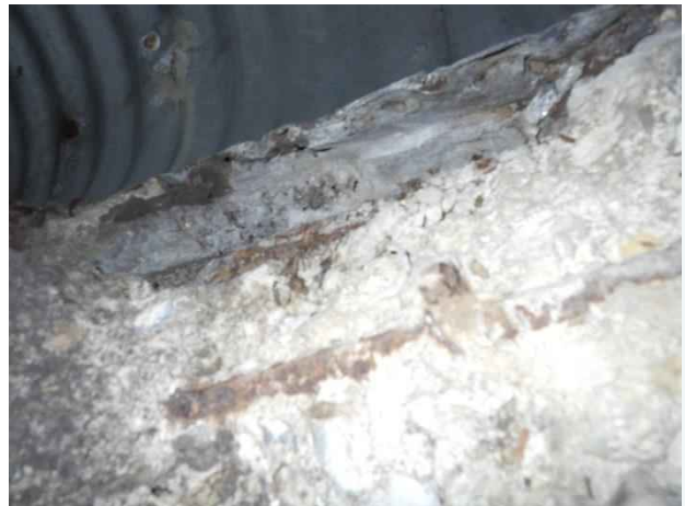
Photo 10. Station 0+85; exposed reinforcement at lateral.
