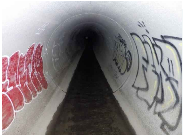
Photo 37. Station 1+25; RCP section of segment was in good condition.
