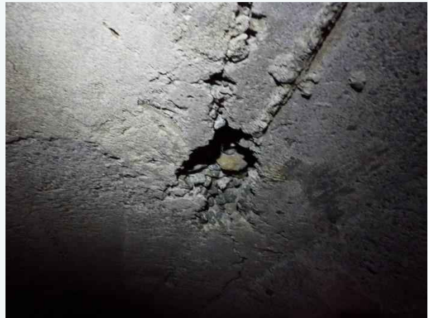
Photo 37. Station 0+14; concrete spalling on arch pipe.
