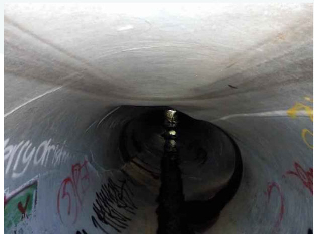
Photo 39. Station 0+70; sag defect on the crown of the pipe.
