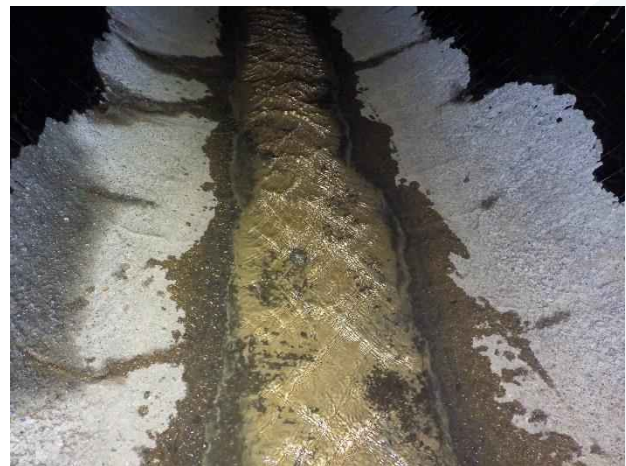
Photo 14. Station 2+00; grout along bottom of pipe.
