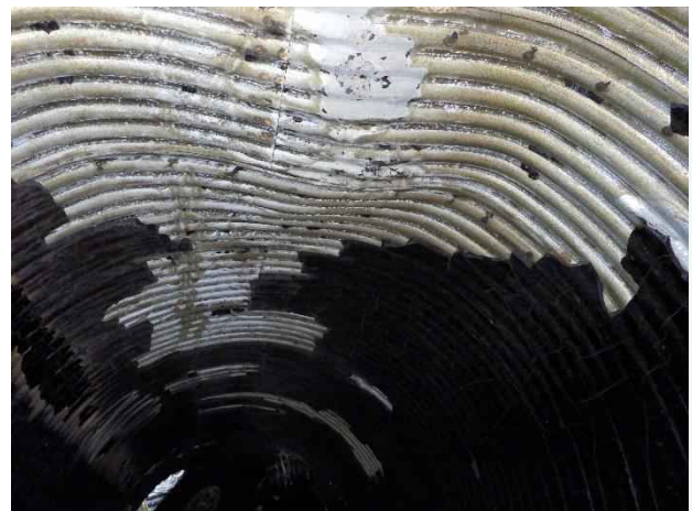
Photo 20. Station 3+54; signs of minor corrosion on deformed bulge.
