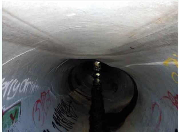
Photo 41. Station 0+70; sag defect on the crown of the pipe.
