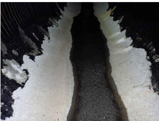
Photo 23. Station 0+80; concrete grout along the bottom of the pipe; typical for segment 1.
