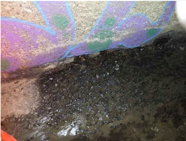
Photo 36. Station 0+14; minor concrete void along the bottom of the arch pipe.
