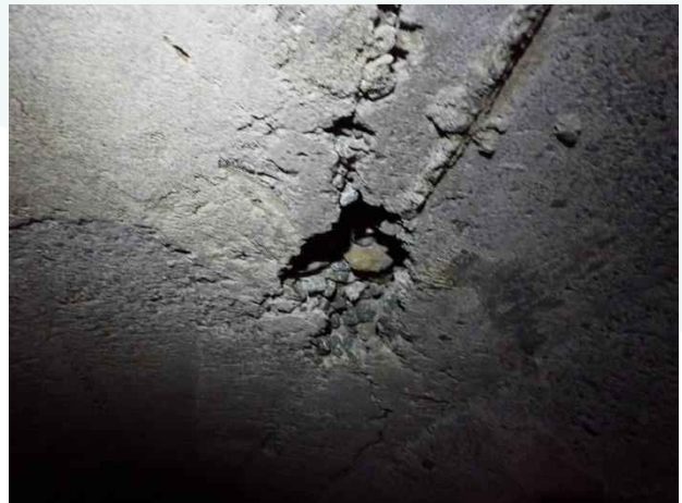
Photo 39. Station 0+14; concrete spalling on arch pipe.
