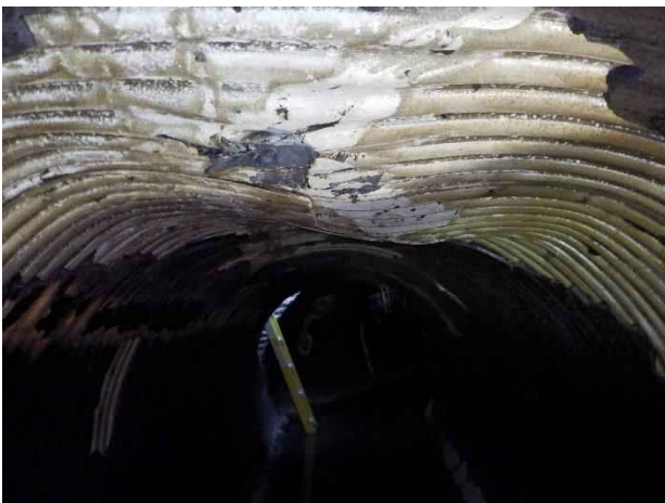
Photo 19. Station 3+54; deformed bulge defect on the crown of the pipe.
