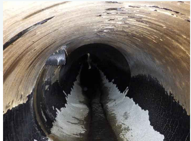
Photo 22. Station 0+80; coating discoloration from 9:00 to 3:00.
