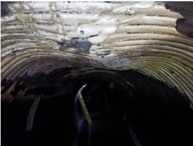
Photo 17. Station 3+54; deformed bulge defect on the crown of the pipe.
