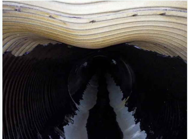
Photo 26. Station 2+05; bulge deformation defect on the crown of the pipe.
