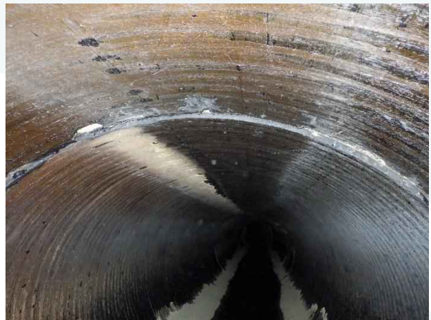
Photo 31. Station 0+46; coating uneven at joint.
