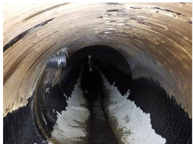
Photo 24. Station 0+80; coating discoloration from 9:00 to 3:00.
