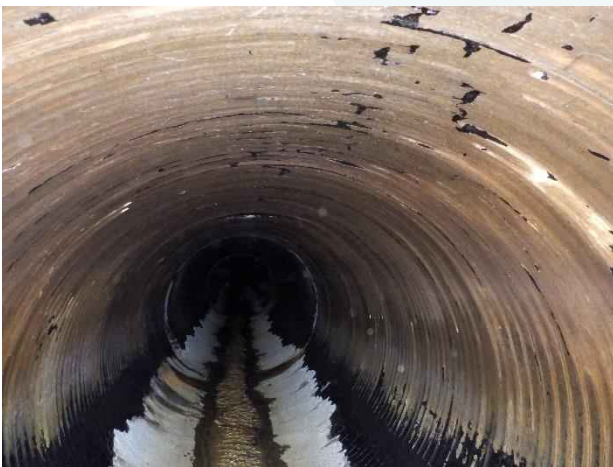
Photo 17. Station 2+00; coating discoloration from 8:00 to 4:00 of pipe.
