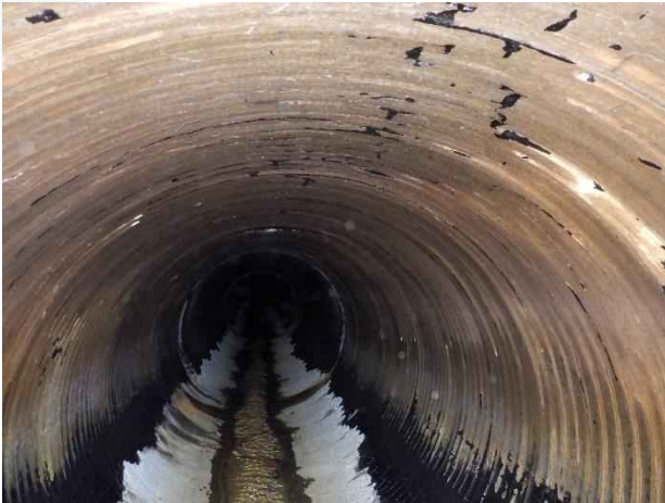
Photo 15. Station 2+00; coating discoloration from 8:00 to 4:00 of pipe.
