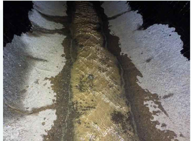
Photo 16. Station 2+00; grout along bottom of pipe.
