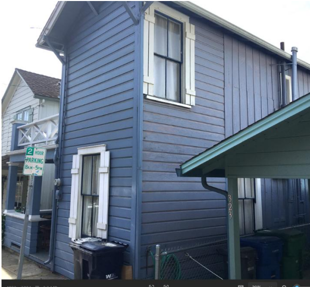
Figure 3: Side elevation demonstrating the horizontal boards on the front elevation, partially wrapping on the side, with board-and- batten to finish.
