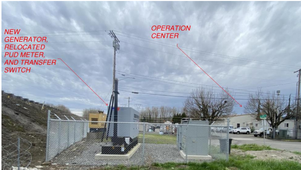
Generator Installation on Polk Street
