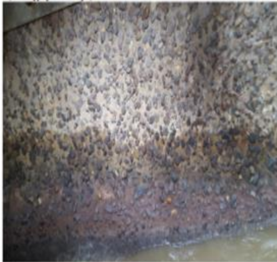
Figures 1-2: Damaged concrete in Headworks
