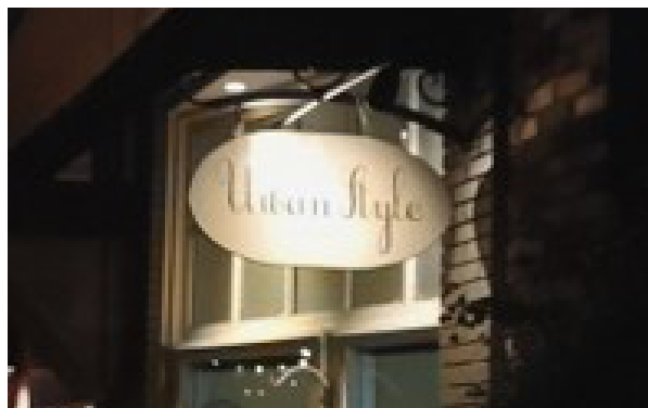
Figure 105. Example of facade fixture where a sign holder with lights on arms integrated into the bracket hold bulbs exactly the right distance from the sign face in Camas, WA [Photo credit: Seanette Corkill]
