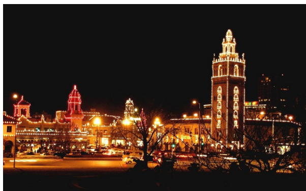
Figure 102. Example of ridgeline and building edge lighting from Country Club Plaza, Kansas City, MO
