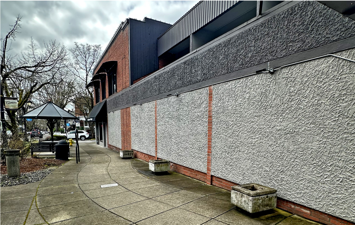
Figure 72. Example of a Blank Wall in Downtown Camas
