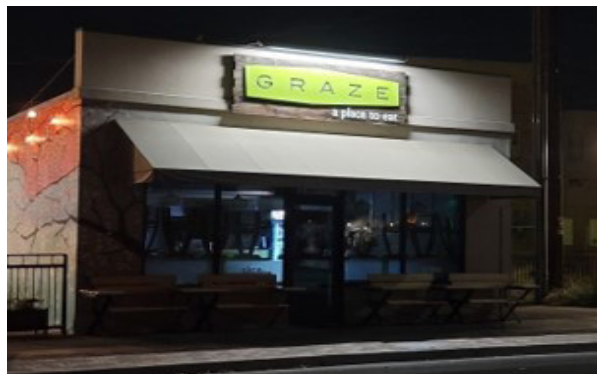
Figure 104. Example of facade fixture where a linear wash of light illuminates a sign in Walla Walla, WA [Photo credit: Seanette Corkill]
