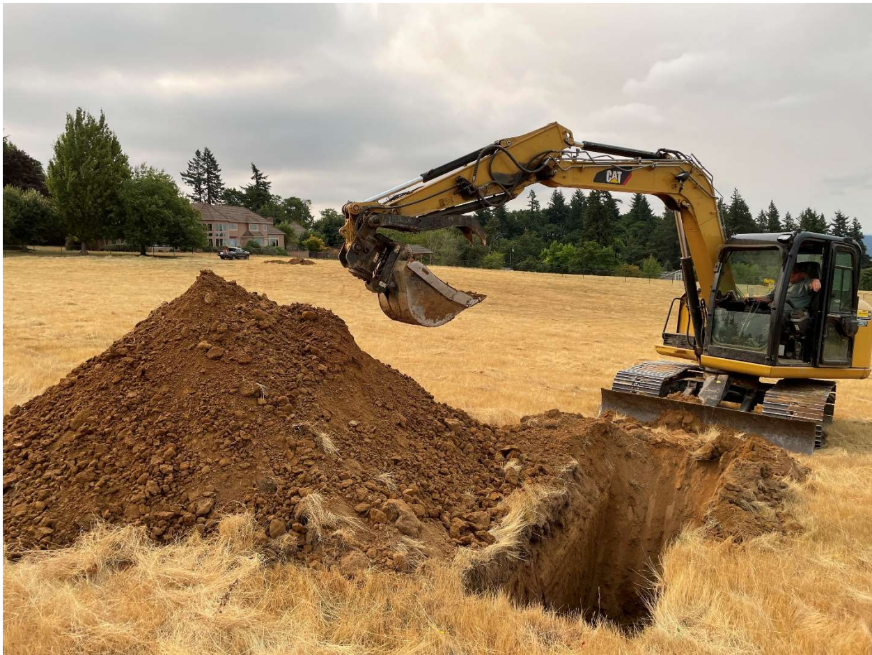
TP-2 Site Area, Facing Southeast
