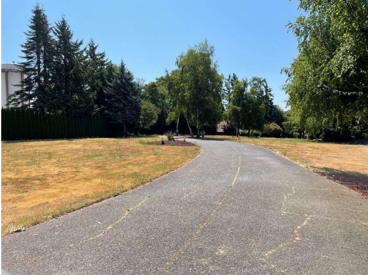
Eastern Site Area, Facing South
