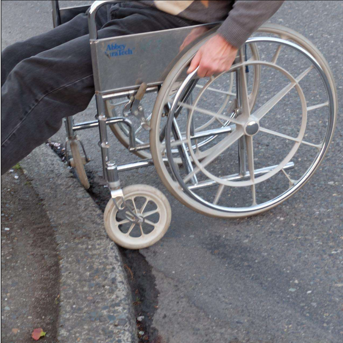
Figure 1: Example of ramp lip of gutter that is a barrier to the disabled
