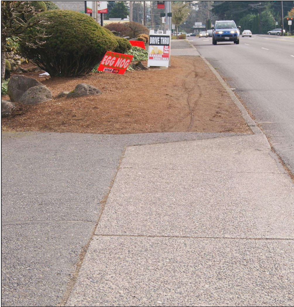
Figure 6: Examples of existing missing sidewalk section
