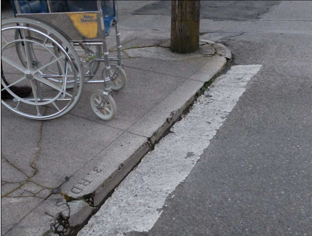
Figure 3: Example of full height curb that is a barrier to the disabled
