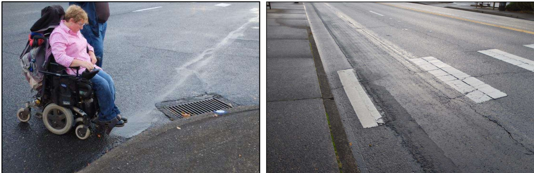
Figure 6: Examples of levels of accessibility experienced during the CAC field tour, such as a missing ramp and a ramp with an outdated design
