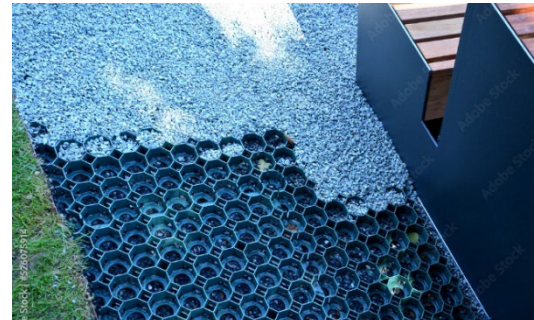
Permeable surfaces should be used in the overall stormwater management plan for developments (Source: © Michal / Adobe Stock)
