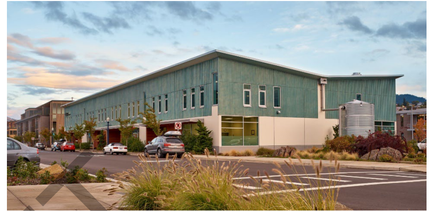
At the LEED Silver Halyard Building in Hood River, OR, rooftop equipment is screened from the street, parking is located behind the building, and a stormwater cistern collects runoff. (Source: Halyard Building 2, robcon.com)
