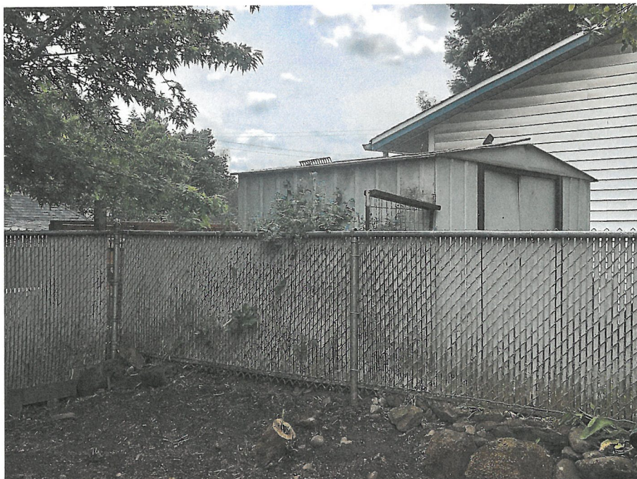
Encroaching shed to southwest of west property line
