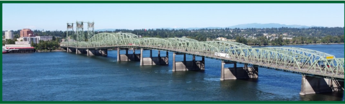
108-year-old I-5 Bridge.
