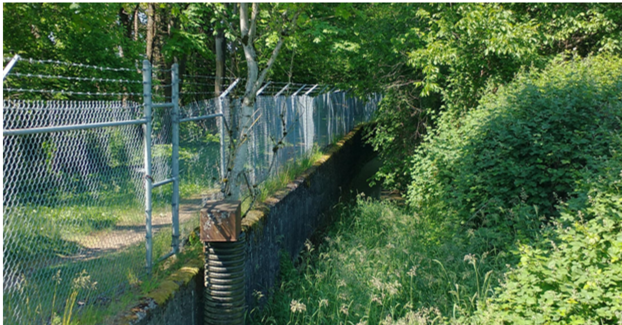
Figure 6. Crown Zellerback Power Ditch
