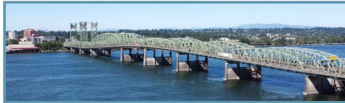
107-year old I-5 Bridge
