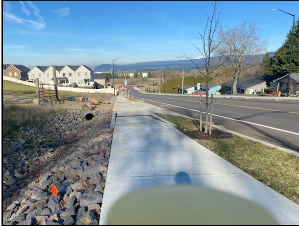
Figure 7: NW Brady Road & Site Access Driveway #1 Looking North
