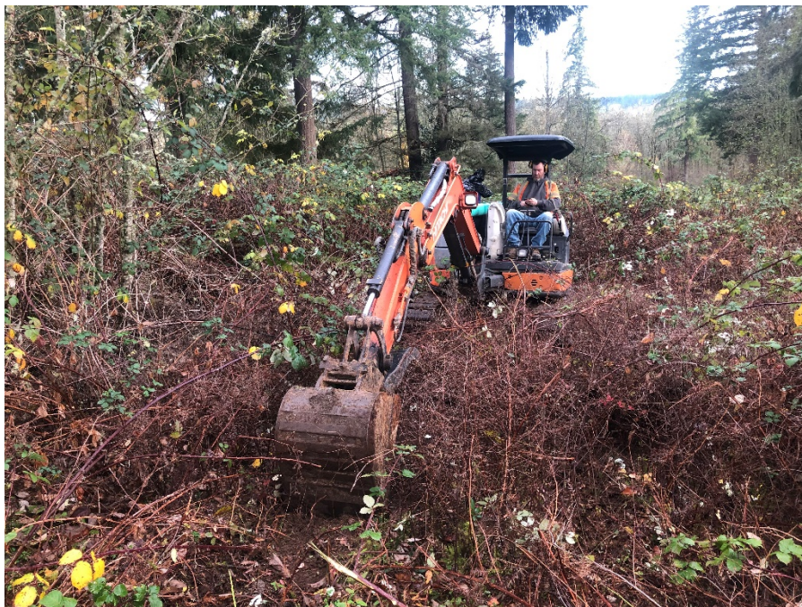
Test Pit TP-8, Facing North
