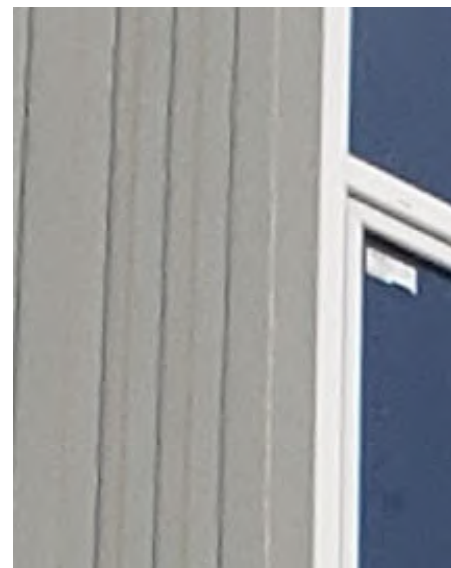
EXTERIOR CLADDING OPT. 2 CEMENTITIOUS BOARD + BATTEN
