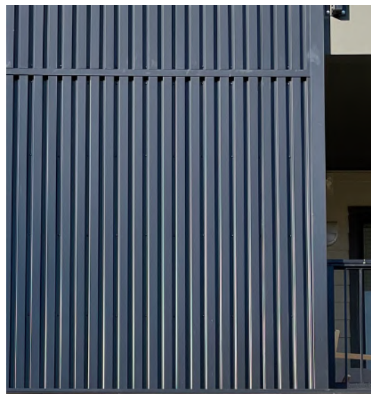
EXTERIOR CLADDING OPT. 1 - METAL PANELS
