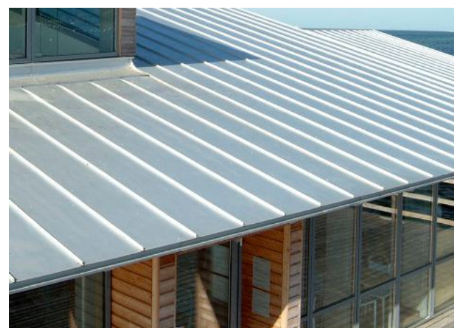
STANDING SEAM METAL ROOF
