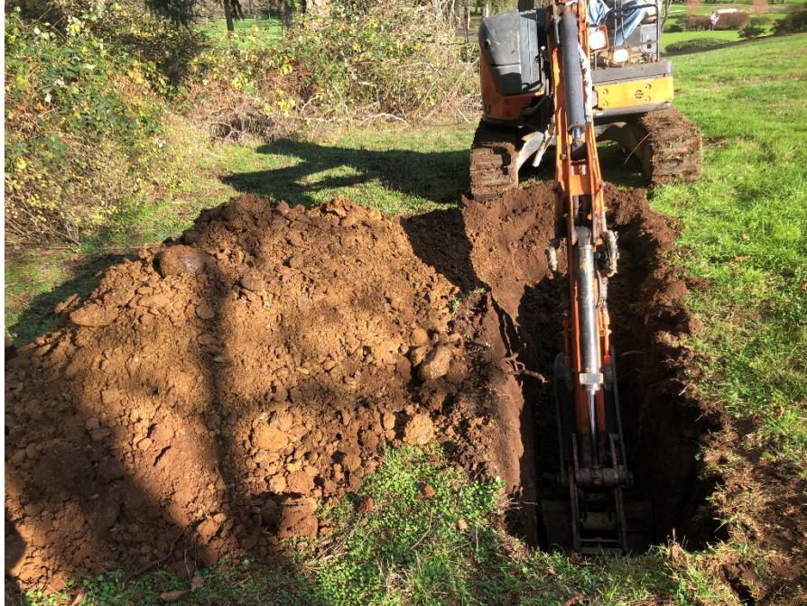
Test Pit TP-7, Facing North
