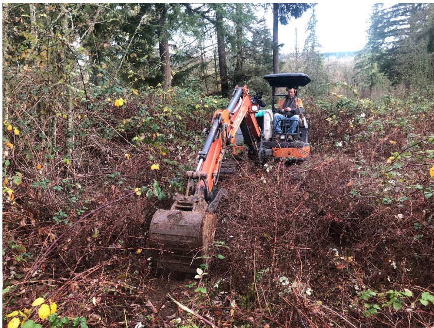
Test Pit TP-8, Facing North
