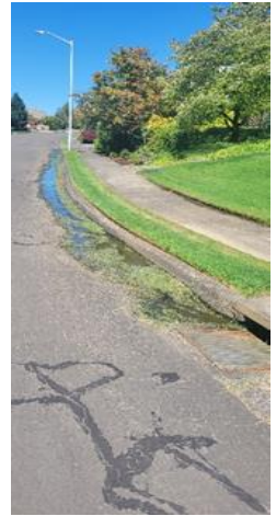
Evidence of underground springs @ 1918 Columbia Summit Dr. - 8/22/2022
