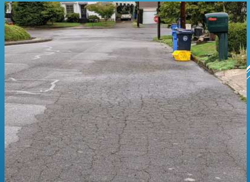
NW 19 TH AVE, LOOKING EAST TO DIVISION ST
