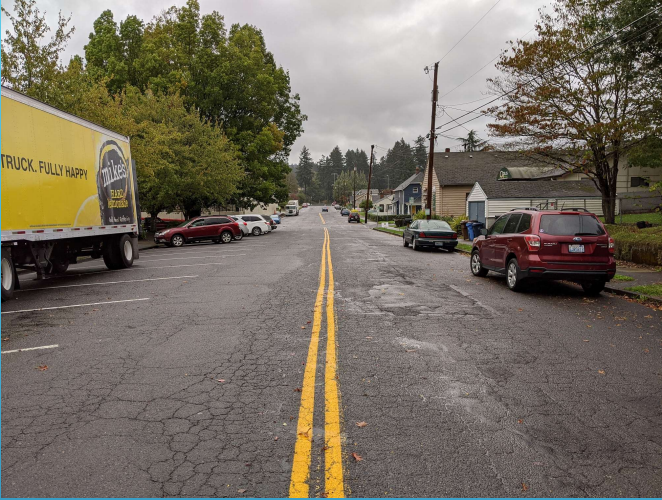
NE 2 ND AVE. AT NE FRANKLIN ST. LOOKING EAST
