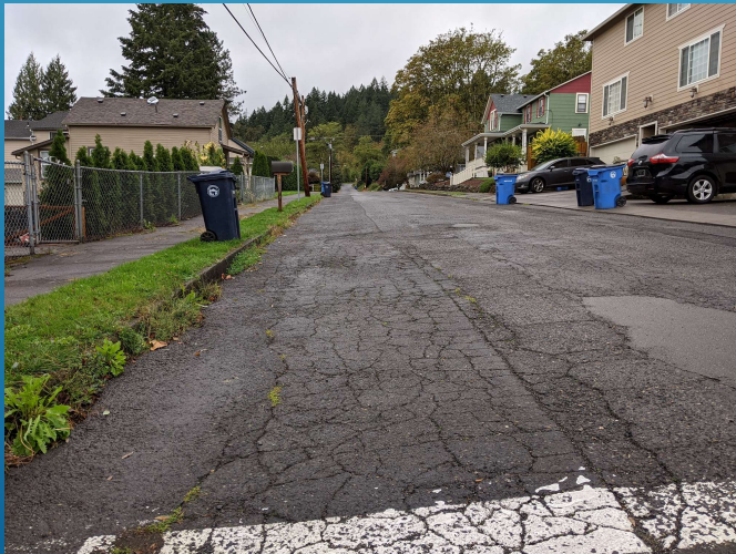
NW 14 TH AVE. AT NW ASH ST. LOOKING WEST
