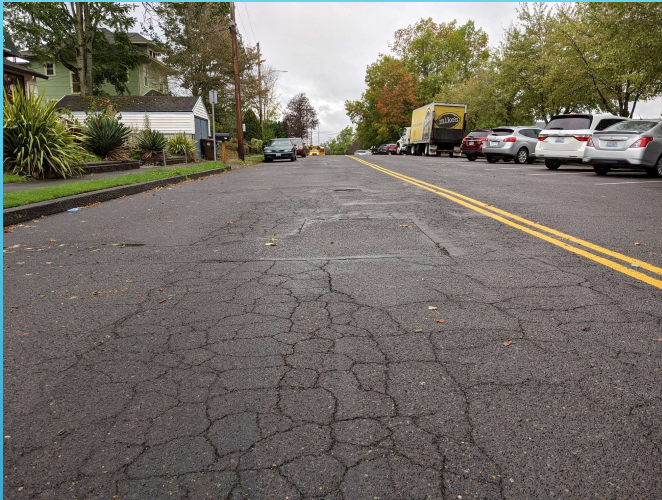
NE 2 ND AVE. AT NE GARFIELD ST. LOOKING WEST
