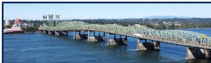
105-year old I-5 Bridge
