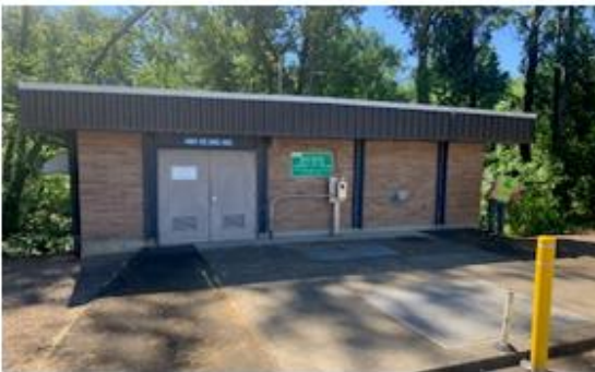
Fig.5: Front of Pump Station
